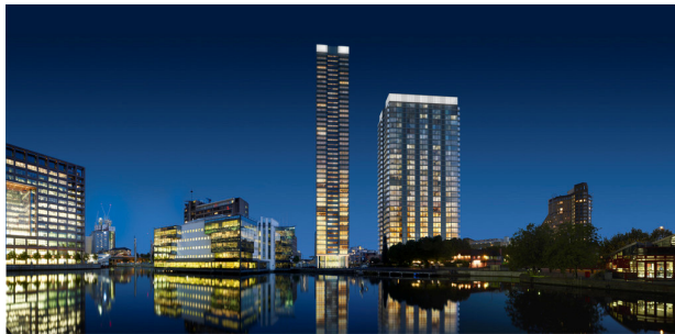
The Landmark East & West Towers, Canary Wharf ©Hayes Davidson
